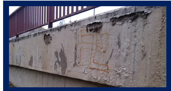
The left-facing swastika near Faraktár street, Source: An Action and Protection Foundation volunteer
